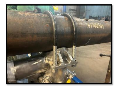
4. Tighten the nuts on the U-Bolts finger tight until the o-ring on the unit is making contact with the pipe.
